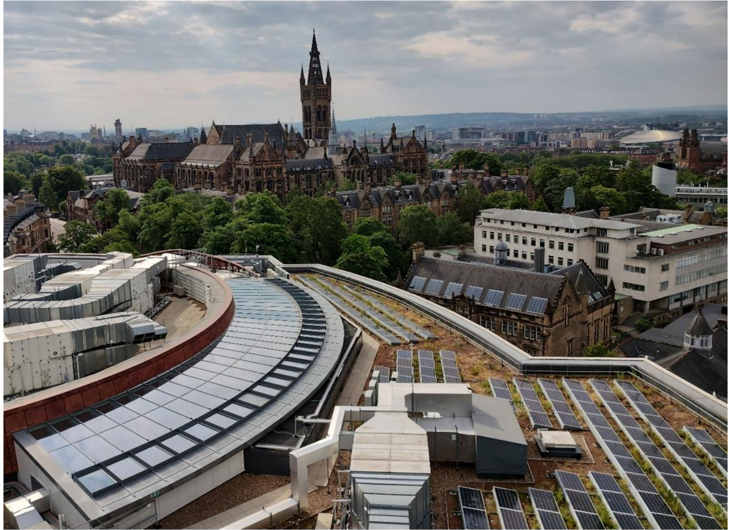
Biosolar PV roof installation at the James McCune Smith Building – power, rainwater attenuation, biodiversity
